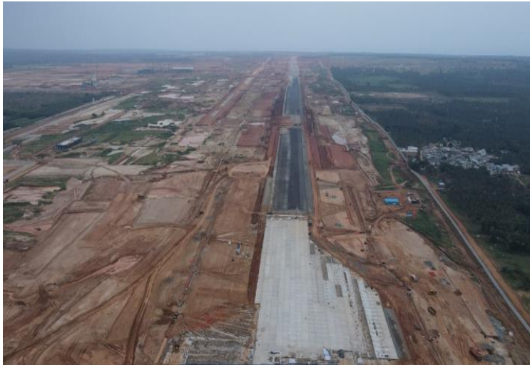
Runway Works Pavement Quality Concrete Layer
